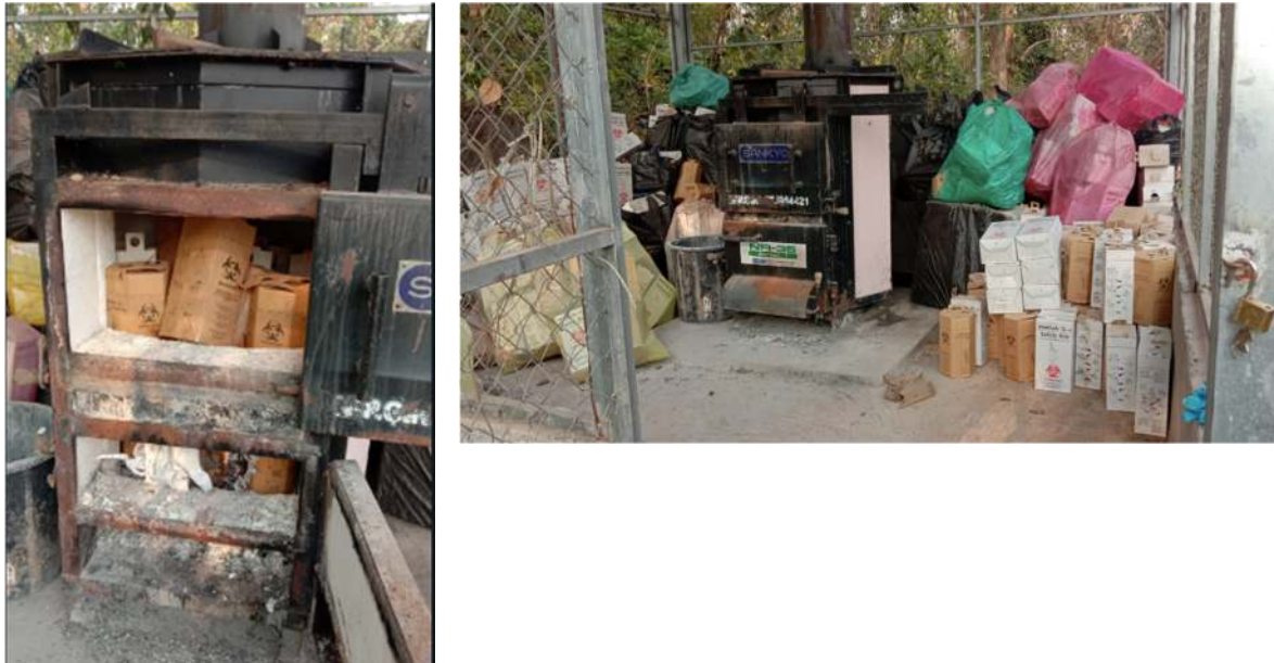
Figure 3: An outdated incinerator has been used for burning disposed syringes delivered from all districts and hospitals in Oudomxay Province
